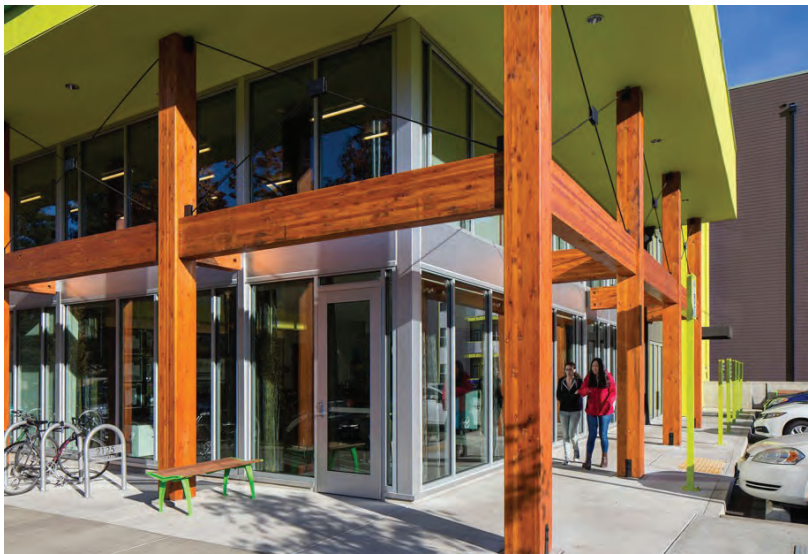
Example of using exposed mass timber structural elements as part of an emerging west coast character (guideline 23). Also includes pedestrian and cycling supportive features such as private sidewalks along the length of the building entry (guideline 57); weather protection (guideline 59); and seating and bike parking (guideline 31).
